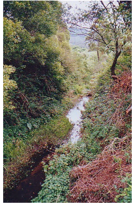
Plate 30: Looking west along Hewitts Creek through Zone 8 showing weed invasion and scouring.
