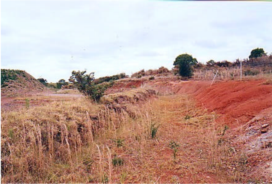
Plate 25: Looking east down line of piped section of Woodlands Creek in Zone 7
