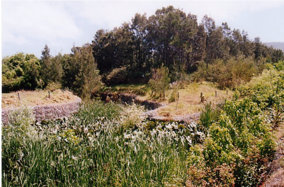
Plate 36: Looking south-west from northern bank of gabioned section Hewitts Creek in Zone 10. Casuarina grove in centre background defines the edge of the remnant swamp wetland of Zone 9. Note weed domination in constructed channel.
