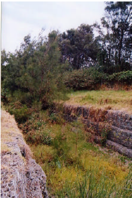
Plate 37: Looking south through constructed gabion diversion channel between Woodlands and Hewitts Creeks. Casuarinas in Zone 9 at background.
